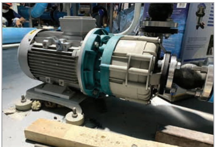
THAILAND. Aquarium ROUTE pump for circulation of seawater for small size pools
