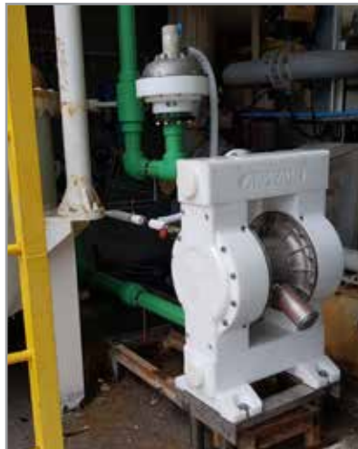
ITALY. Chemical plant QUANTUM (DDQ 160) pump for unloading HF from reactors at 160°C. MISTRALsolid (DDM 300 PE1000) pump with PE1000 pulsation dampener for the circulation of acids at 60°C.
