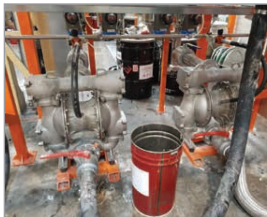
ITALY. MISTRAL (DDM 400 AISI316I) pumps for loading oily water.
