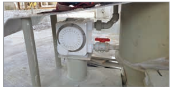
ITALY. Chemical plant QUANTUM (DDQ 160) pump for unloading HF from reactors at 160°C. MISTRALsolid (DDM 300 PE1000) pump with PE1000 pulsation dampener for the circulation of acids at 60°C.
