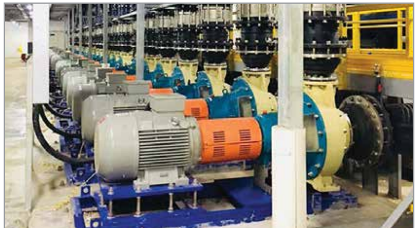
CHINA. Hotel Resort with aquarium and swimming pools - for the circulation of seawater to the various pools
