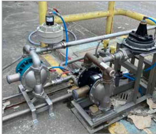
FRANCE. Gypsum production plant ASTRAevo (DDE 400 AISI316L) pump for liquid gypsum.
